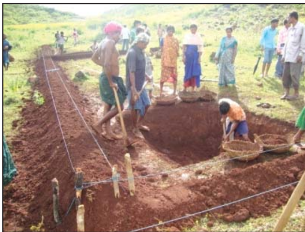
Ongoing 30 x 40 model land development work
