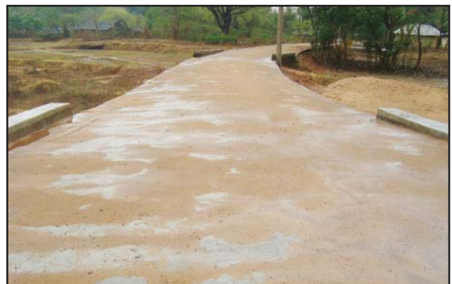
Construction of C.C. Road at village Ghodabundha
