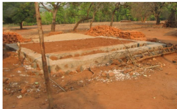
IAY construction work in progress under convergence at Keonjhar
